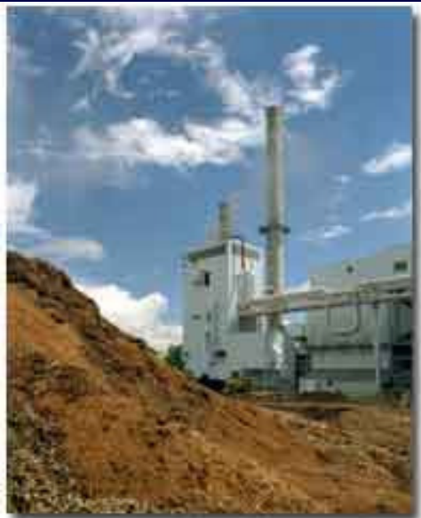
Biomass Power Plant - Photo credit: U.S. Department of Energy, Energy Efficiency & Renewable Energy Network (EREN)
